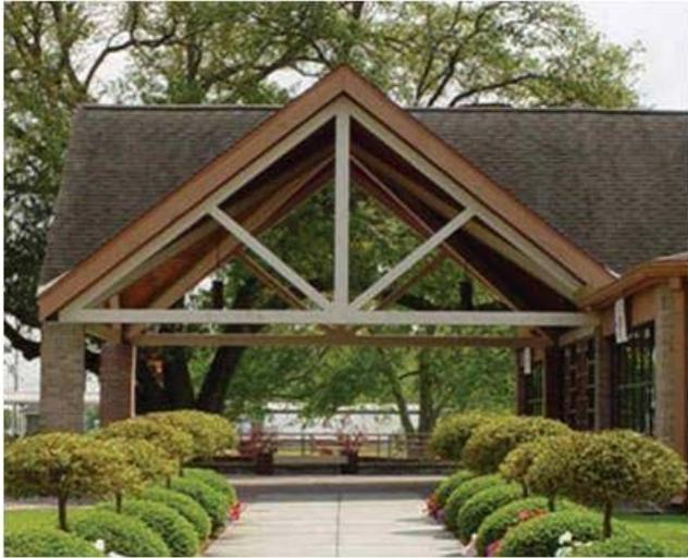
Trusses are commonly used to support roofs.
