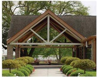
Trusses are commonly used to support roofs.
