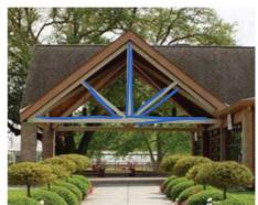
Trusses are commonly used to support roofs.
