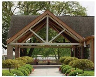
Trusses are commonly used to support roofs.
