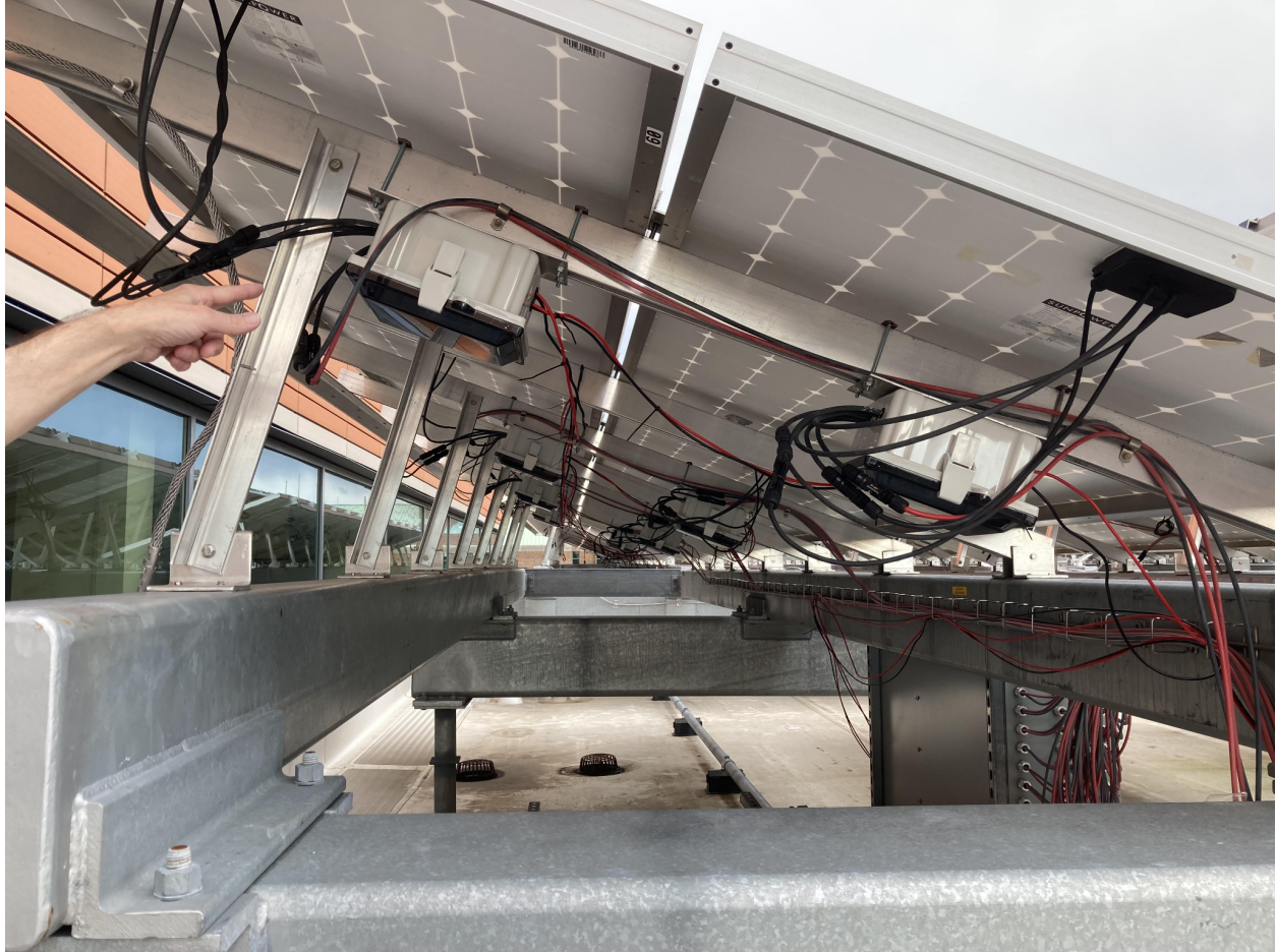
Figure 8: Mounted Attaboxes on the Solar Panels (Roof of ECEB)
