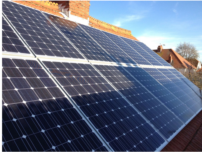
Fig 3. Image of a partially shaded solar panel array [8]
