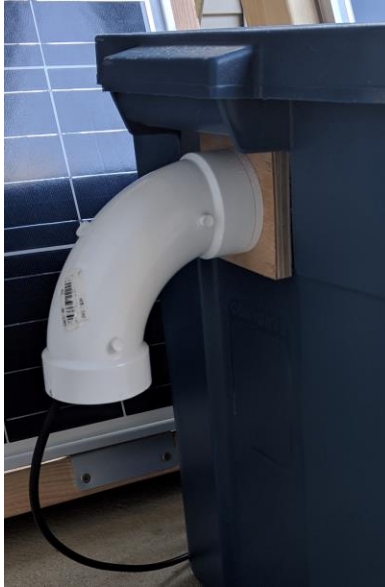
Figure 13. 90 Degree PVC Elbows for Solar Panel Wire Inlets
