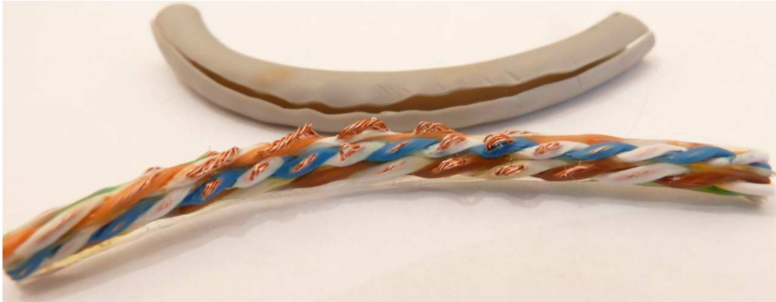
Melted cable (electrical short)
