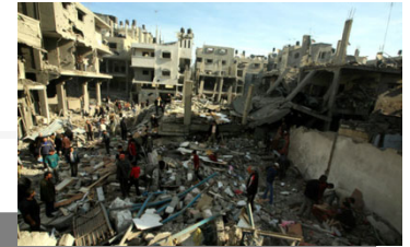
Collapse on Park Ave.
