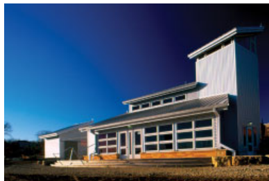
Zero-energy Building: Science House at the Science Museum of Minnesota
