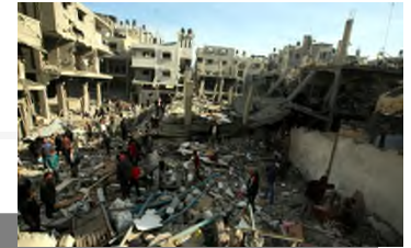
Collapse on Park Ave.
