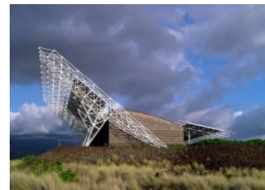
Hawaii Gateway Energy Center
